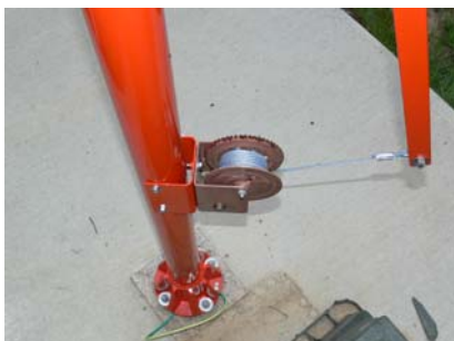
Figure 2.5. L-806 Windcone with a Center-hinged Pole.
